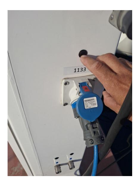
Your ship is **now connected.** You can now use the electricity from your **personal account**. To log out, you can either **hold the** card and **press** the button or **remove** the plug, which **will automatically disconnect** it.
